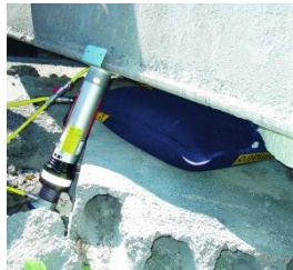
Follow -up shoring
