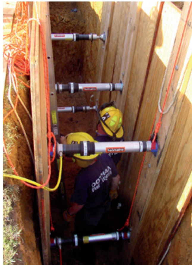
Trench shoring with pneumatic Auto-lock struts.
