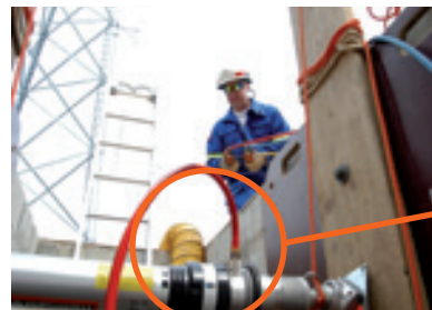
The Auto-lock system enables remote shoring.
