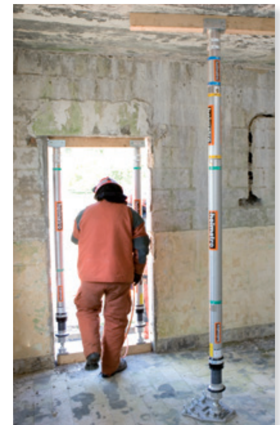
Shores combined with timber to protect the access and exit route of a collapsed building.
