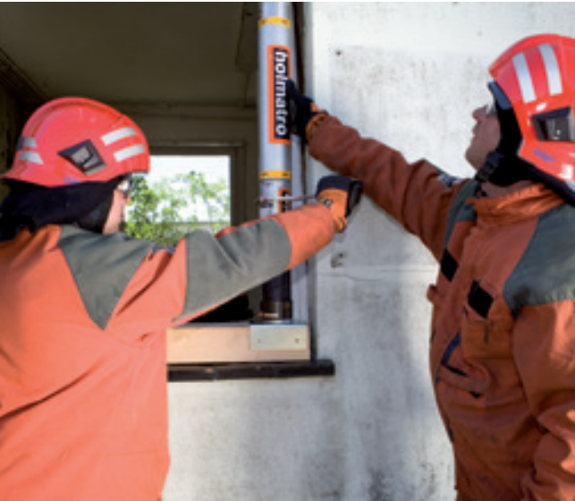
Manual threaded type strut used to shore a window. It can be secured with the help of a hook wrench (see image below).
