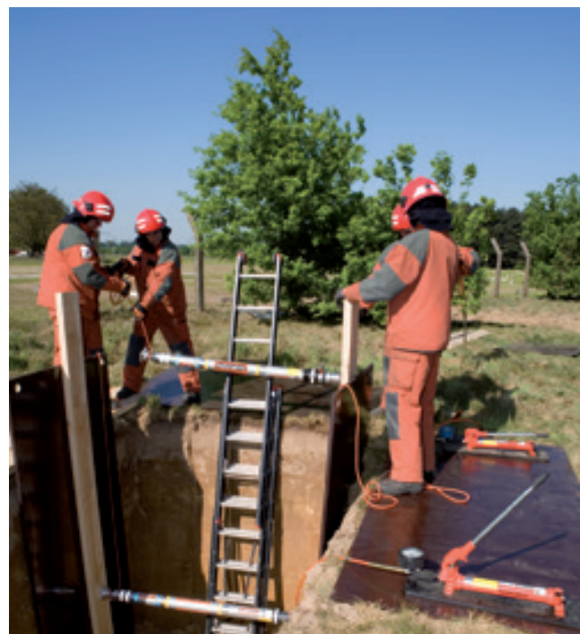
Hydraulic Auto-lock struts used for remote shoring.
