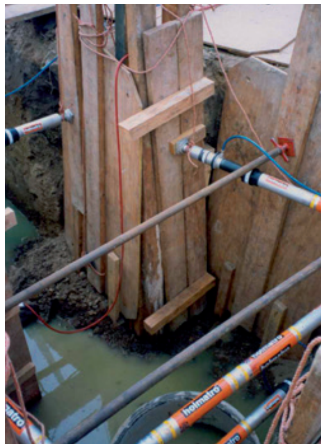
Pneumatic Auto-lock struts positioned in a trench.
