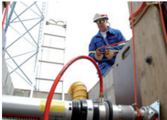
Remote shoring of a trench.
