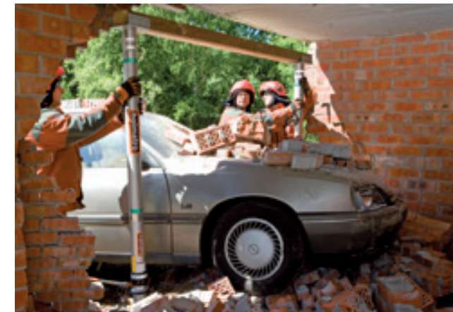
Positioning two shores with beam support heads and a beam, to stabilize a building. The hydraulic Locknut struts will be carefully extended by means of a hand pump.
