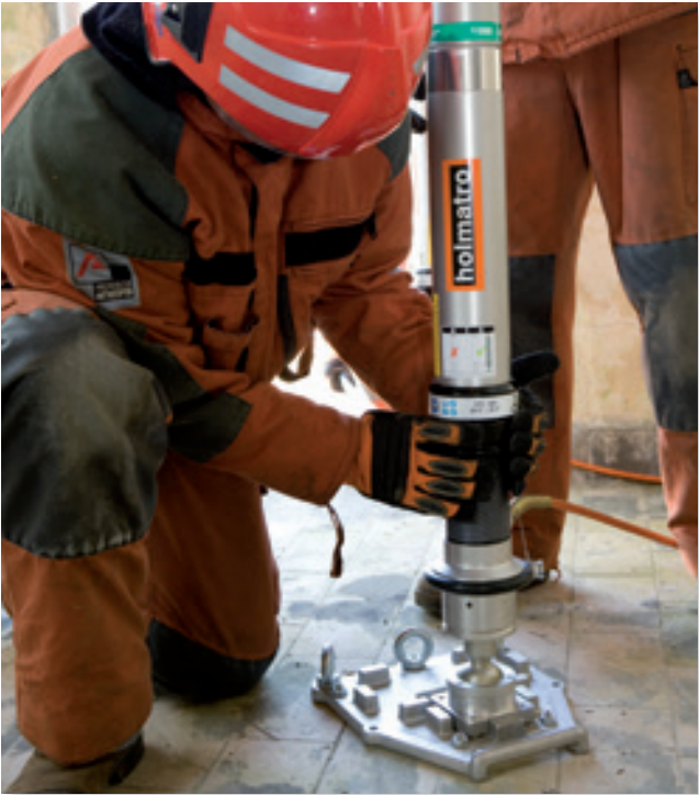
Pneumatic Locknut strut used as a manual strut to shore a building.
