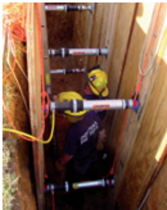
Trench shoring with pneumatic Auto-lock struts.
