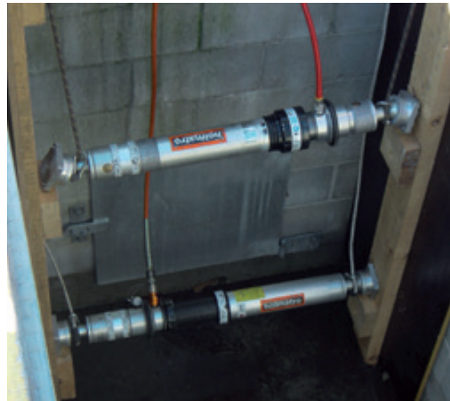
Remote shoring with Auto-lock struts.
