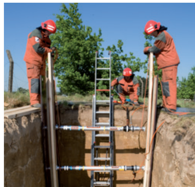
Remote shoring with hydraulic Auto-lock struts.
