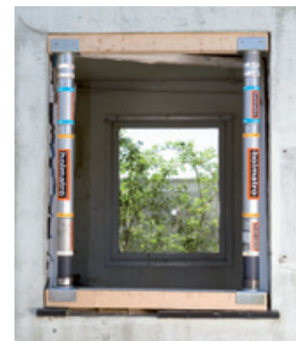
Manual struts with extensions, beam support heads and timber to stabilize a window.
